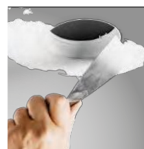
skimmed into plasterboard ceiling (trimless)
