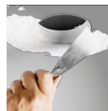
skimmed into plasterboard ceiling (trimless)
