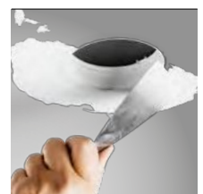
skimmed into plasterboard ceiling (trimless)
