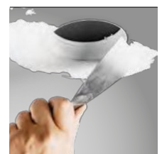
skimmed into plasterboard ceiling (trimless)
